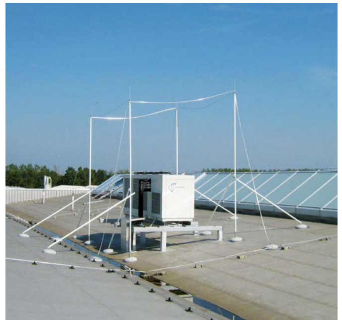
Figure 14: Catching system mounted on insulated load-bearing elements IZ045
